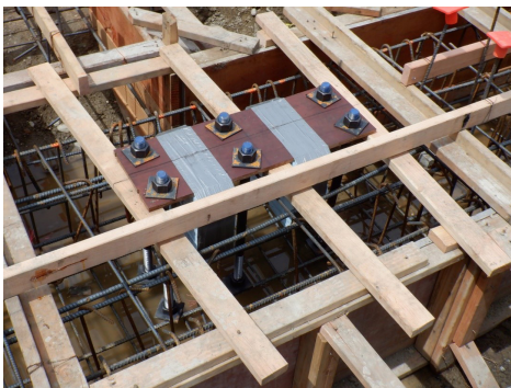
Detail of footing construction for Arlington High School classroom addition
